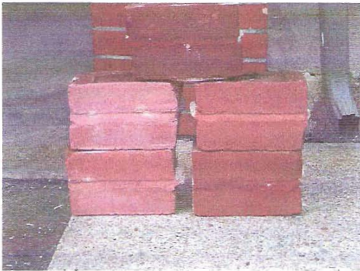
Freshly painted mock-ups February 2005
